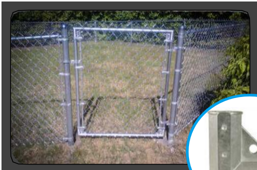
Gate corner uses for attaching gate corners
