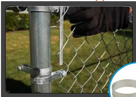
Tension band reinforces chain link fence
