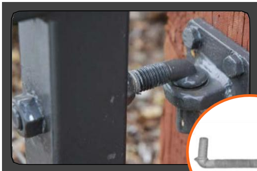
J-bolt hinge connects post to the wall
