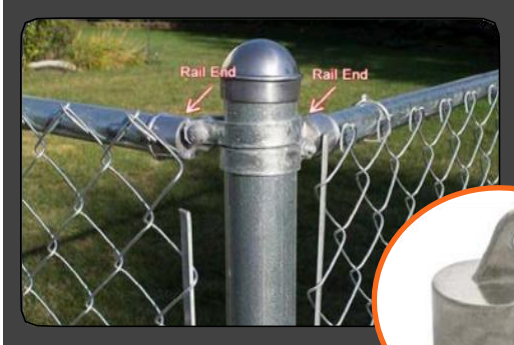
Rail end fix the horizontal post
